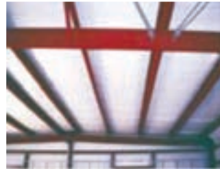
Roof & Wall Insulation
